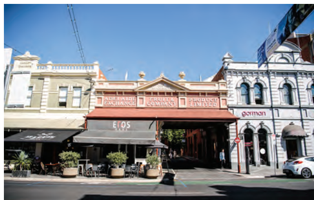
Heritage shop frontages
